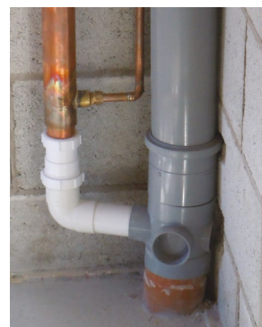
With Waste Water Heat Recovery, it is important to match the correct type and application to the heating system.
